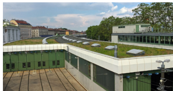
Plants on buildings can play an important role in cooling urban landscapes
